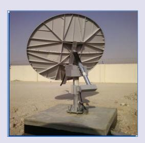
For tracking system we offer you two option, DVD tuner card and beacon receiver. DVB tuner card can use for just Ku-Band antenna. But beacon receiver is fully compliant for Ku-Band and C-Band Antennas.
